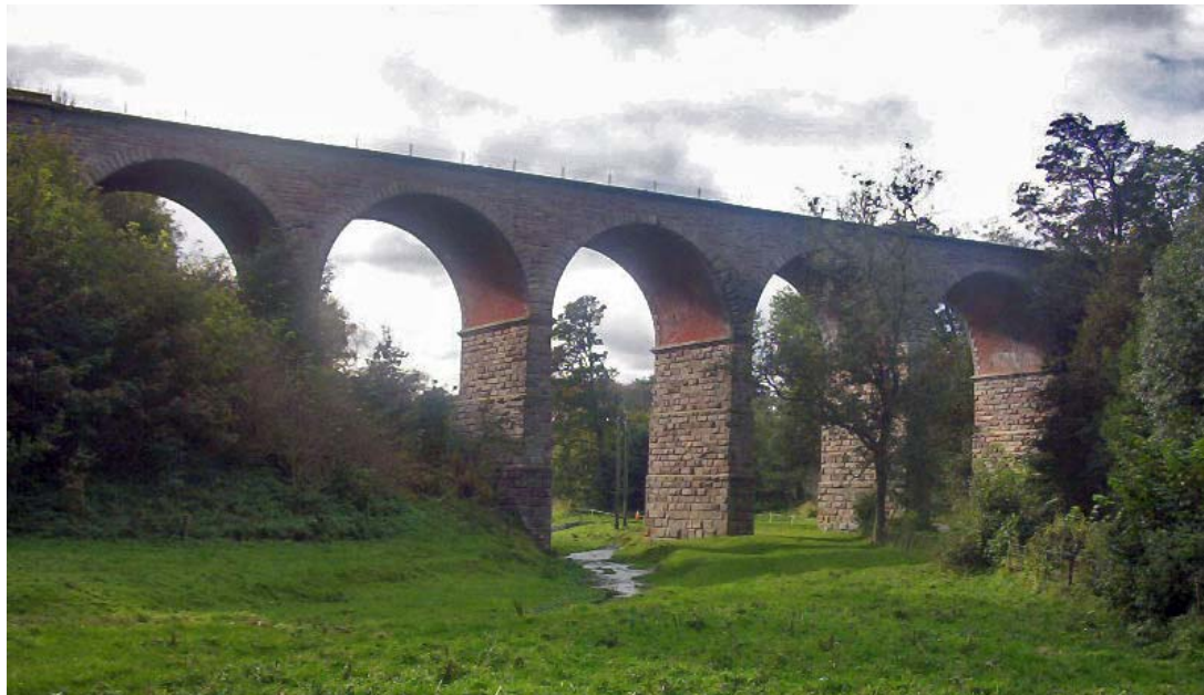
Duddo Burn Viaduct, Northumberland
