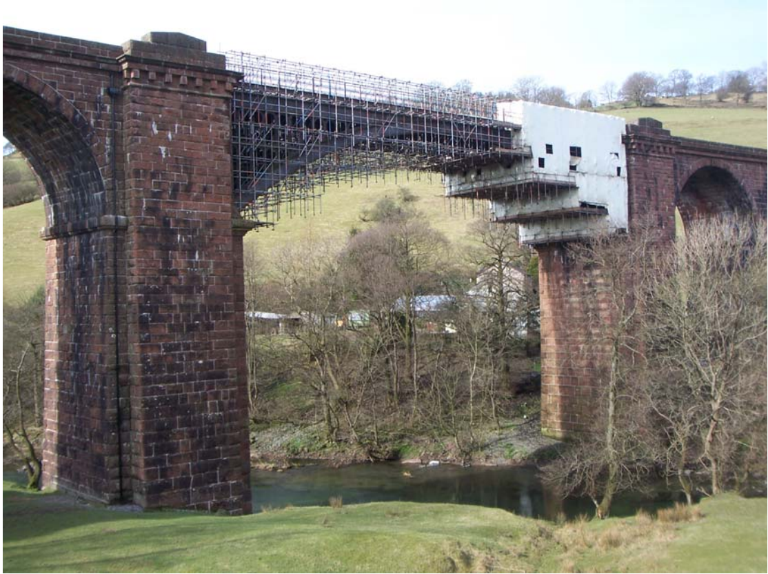
Lune Viaduct, showing work underway
