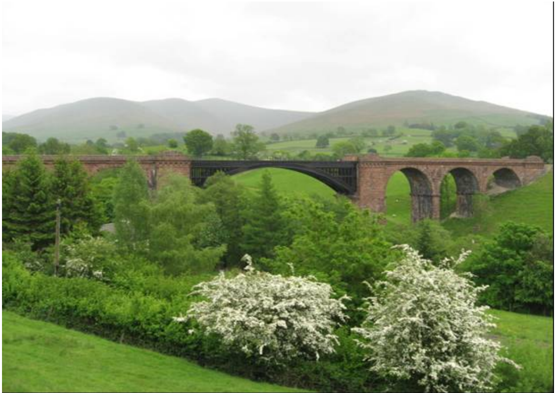
Lune Viaduct, following completion of work
